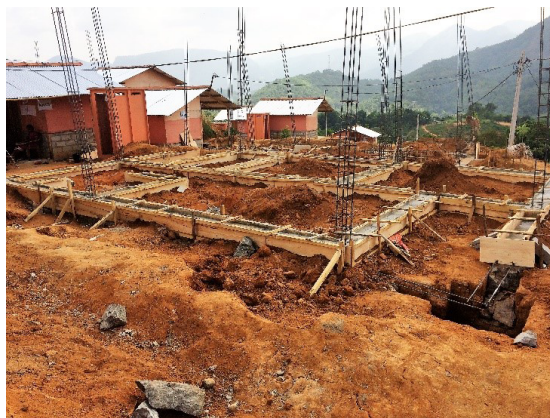
Fig 5(b): Proposed disaster resilient and mitigation building foundation
