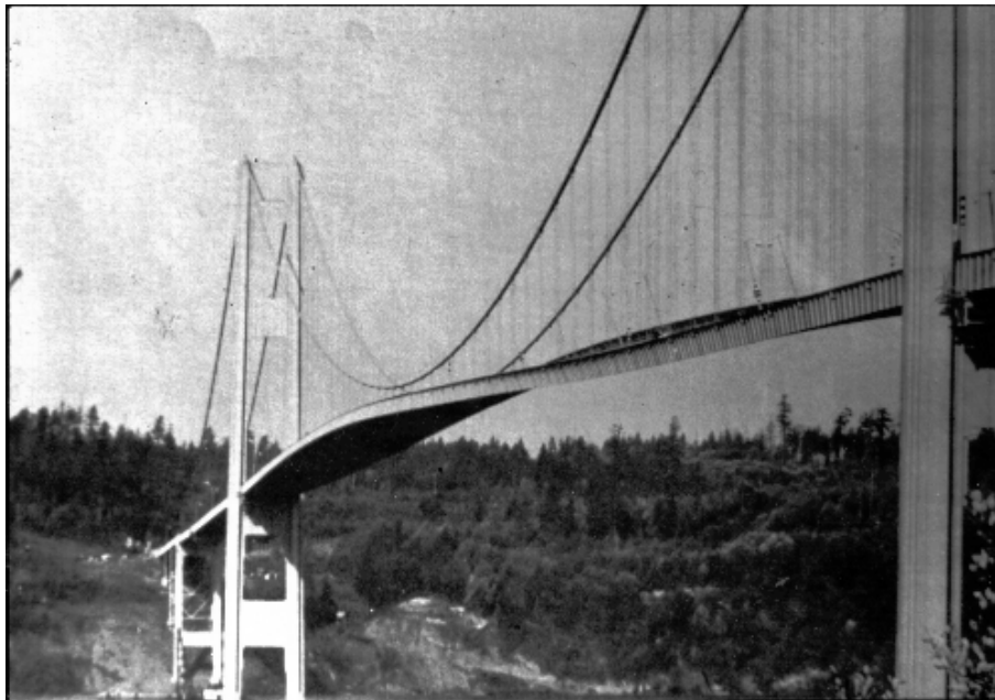
Fig. 4.1 Tacoma Narrows bridge minutes before collapse. Figure courtesy of Wikipedia.
